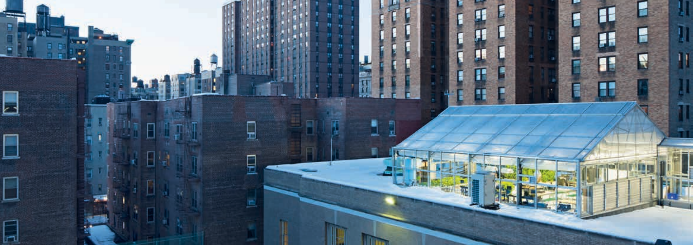
Rooftop Greenhouse, Manhattan School for Children, New York City, USA
