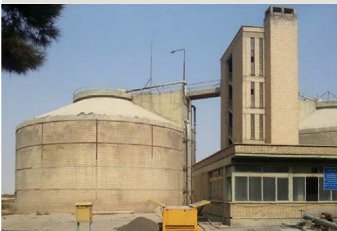
Wastewater Treatment Plant Isfahan North, digester Phase 1.
