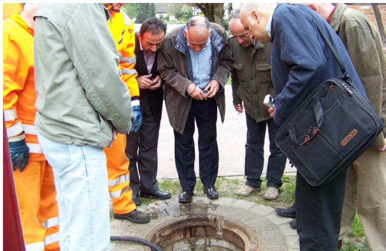
Visit of a sewer shaft for vacuum drainage in Brandenburg.
