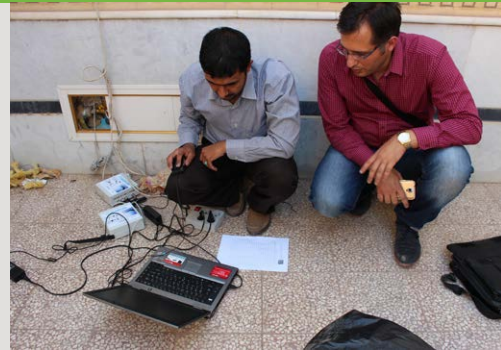
Installation of DEMAPLAN measuring devices.
