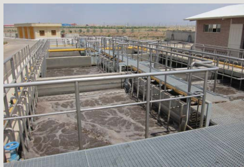
Wastewater treatment plant Moorche Khort.
