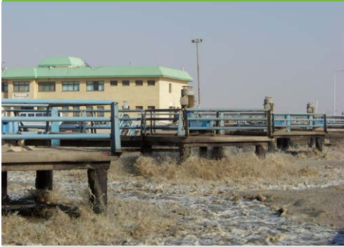
Isfahan North Wastewater Treatment Plant.
