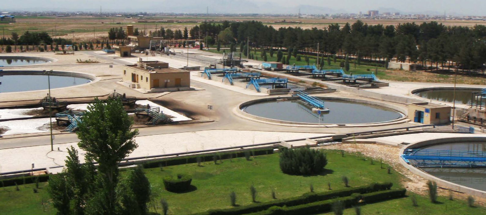
Isfahan North Sewage Plant.
